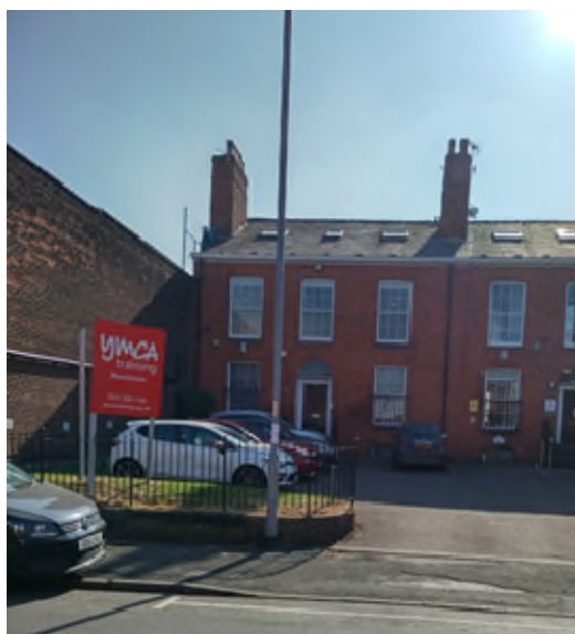
Fig. 2 – Views of the site from Manor Street
