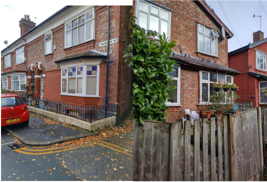
Fig.1 – Views of the front and rear of the application property
