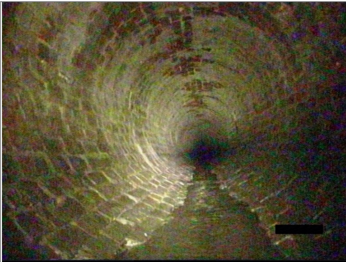
Start node type, manhole, reference MH2
