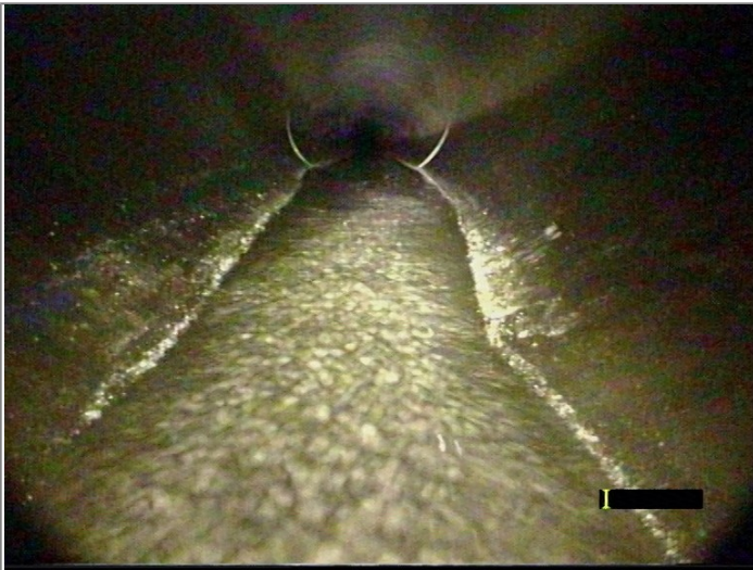
Start node type, manhole, reference MH1
