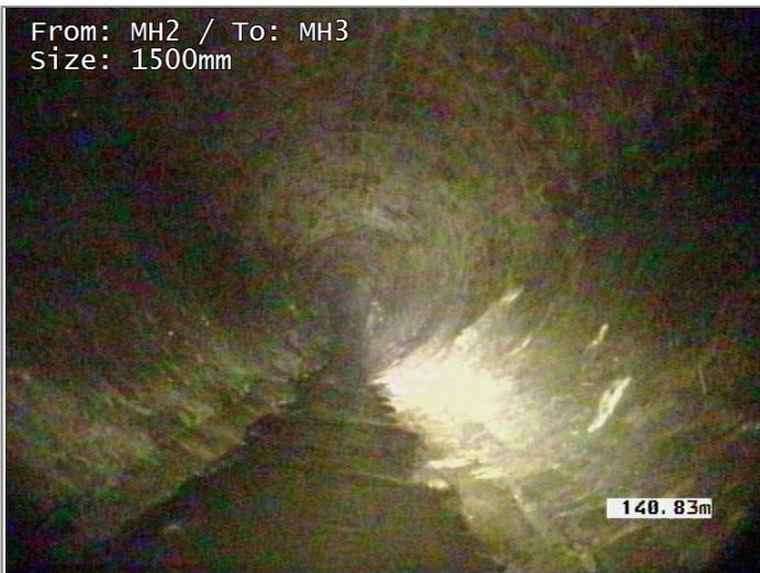
Survey abandoned - Remark: OUT OF CABLE OVERLAP REQUIRED
