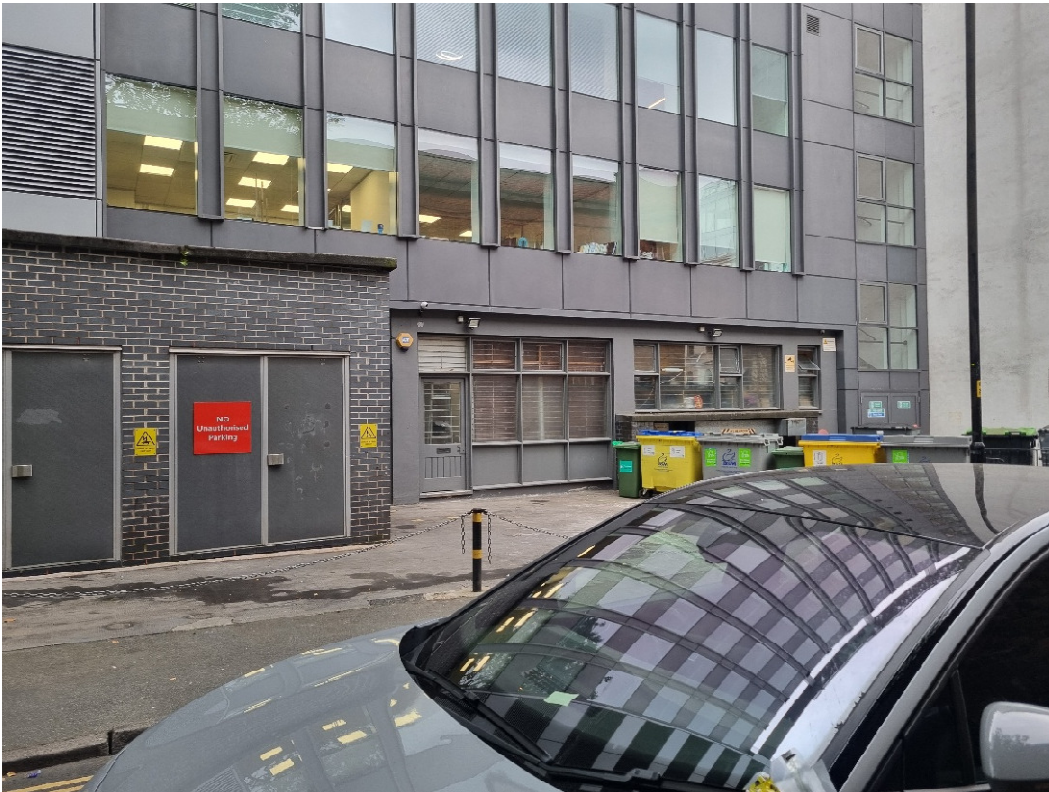
RIGHT HAND SIDE OF EXISTING SUBSTATION ON BOOTLE STREET
