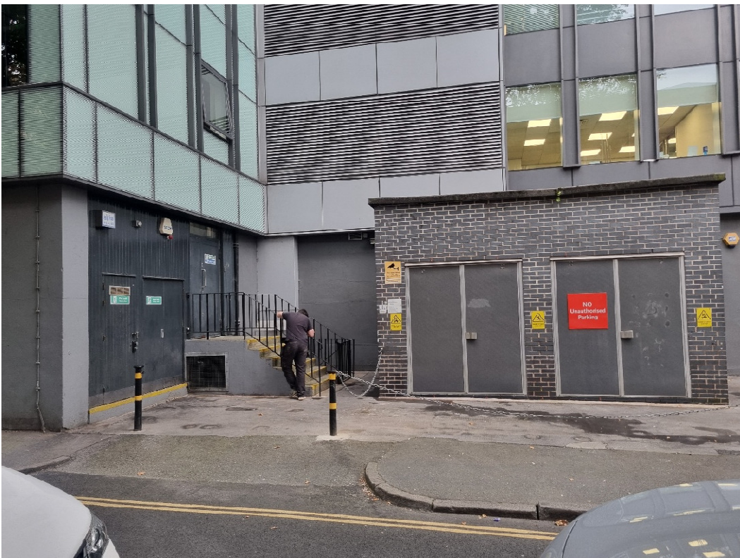
EXISTING SUBSTATION ON BOOTLE STREET
