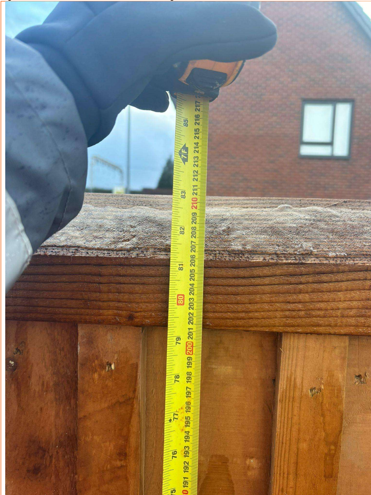
Figure 3 Installed barrier at Plot 9 - height
