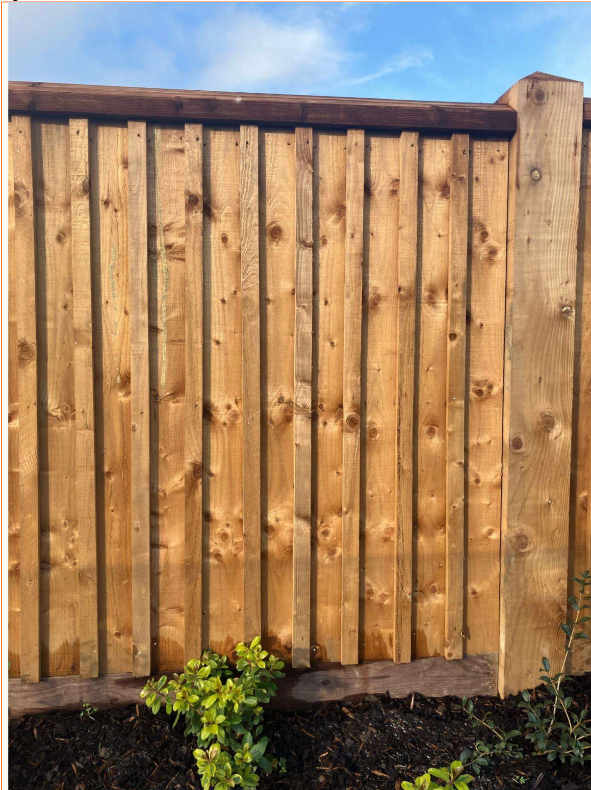
Figure 2 Installed barrier at Plot 9
