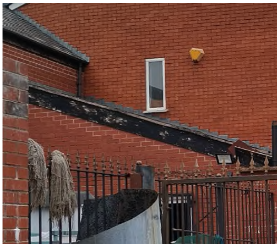
Fig.3 – Window in the side elevation of 2 Mitre Road
