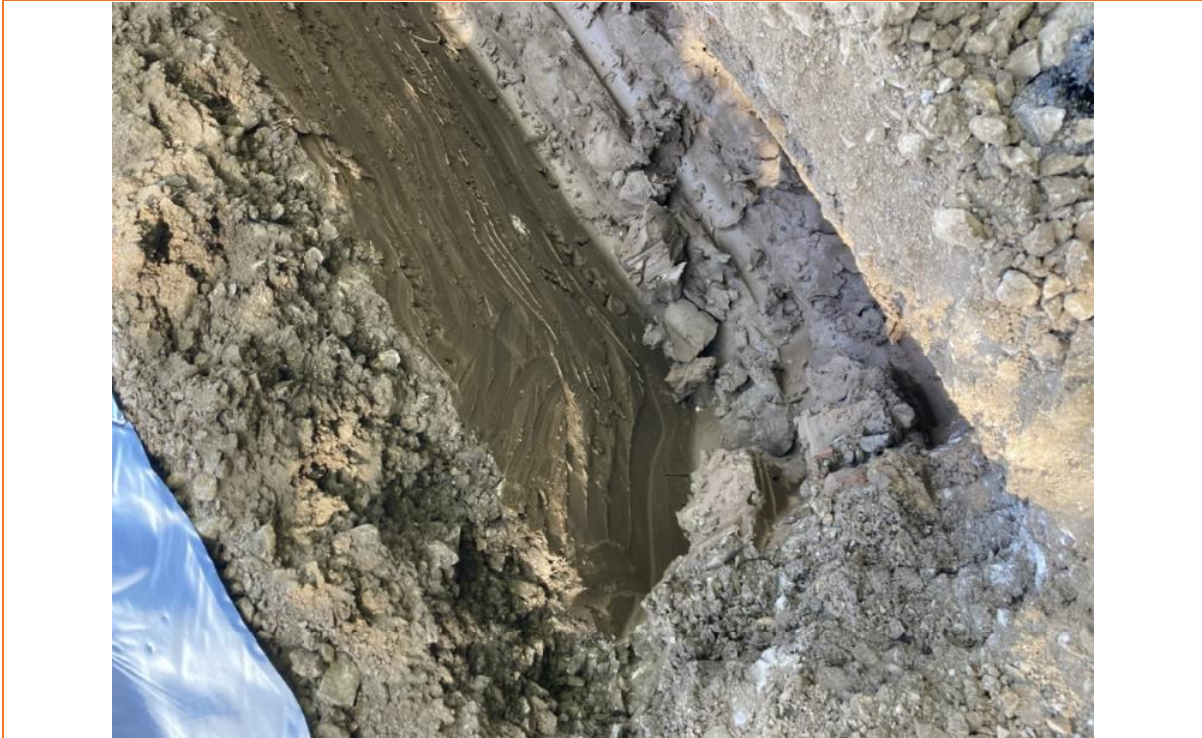
Plate 2 Trial Trenching TS101
