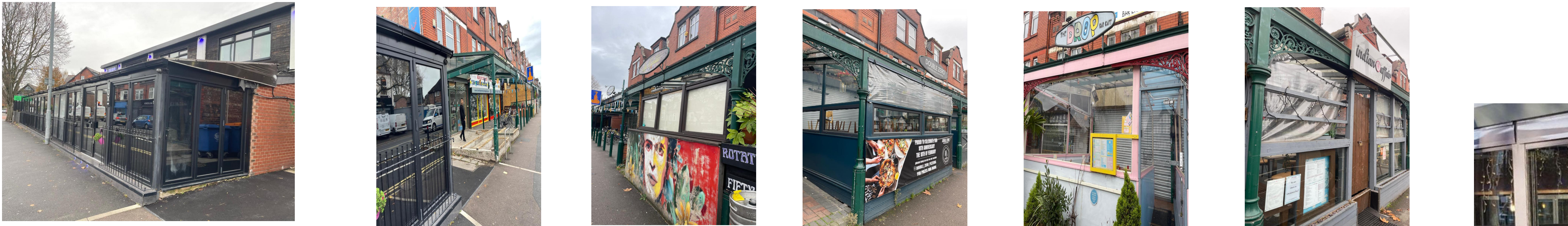
IEWS OF ADJACENT PROPERTIES ALONG BARLOW MOOR ROAD
