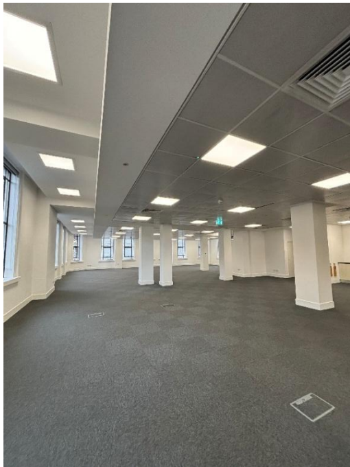
Figure 29: View from the centre of the floor toward the Atlas Chambers building. Source: site visit, October 2025.
