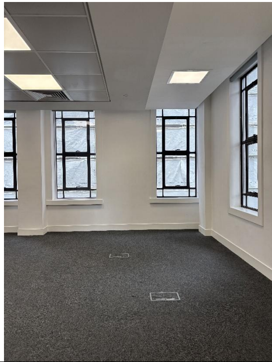
Figure 28: Existing non-original window detail. The fenestration detail is consistent across the floor. Source: site visit, October 2025.
