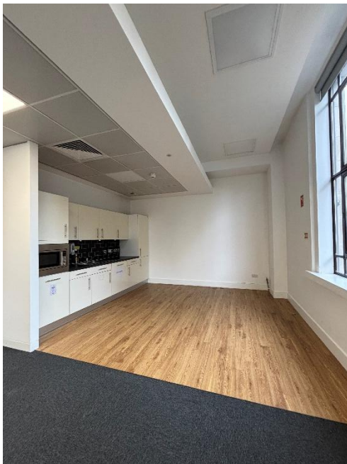
Figure 21: View of the existing kitchen to the right of the floor plate. The existing double-dropped ceiling is shown in detail in this image. Source: site visit, October 2025.
