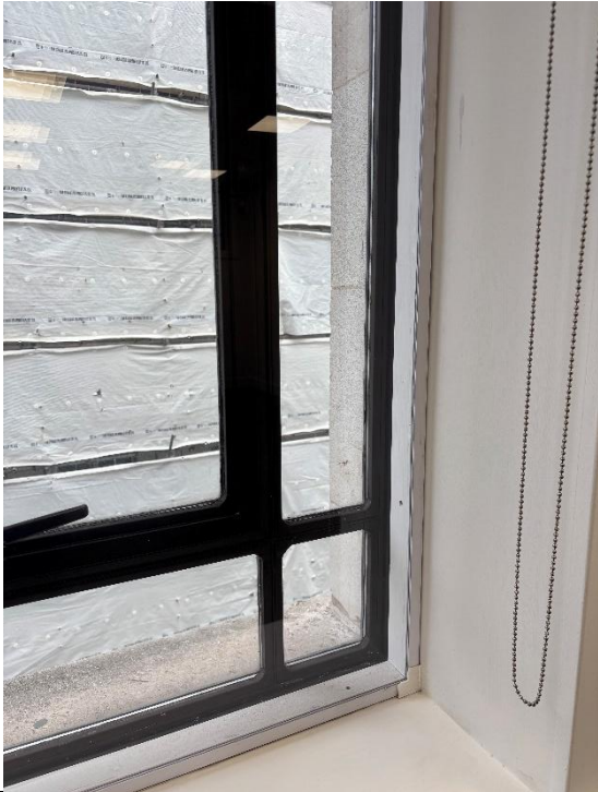
Figure 27: One pane of secondary glazing has been installed along the Brown Street elevation of Atlas Chambers. Source: site visit, October 2025.
