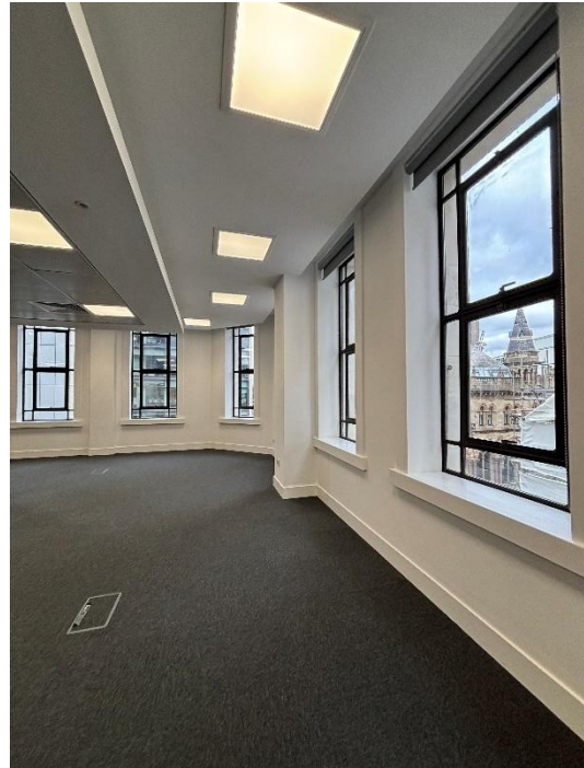
Figure 26: View toward the Atlas Chambers external elevation showing the corner fenestration pattern. Source: site visit, October 2025.
