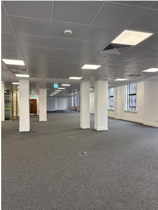
Figure 25: View from the left-most end of the floor looking into the interior. Modern meeting rooms have been installed to the left-hand side of the image, and the original columns have been boxed in. The dropped ceiling is most evident in this view. Source: site visit, October 2025.
