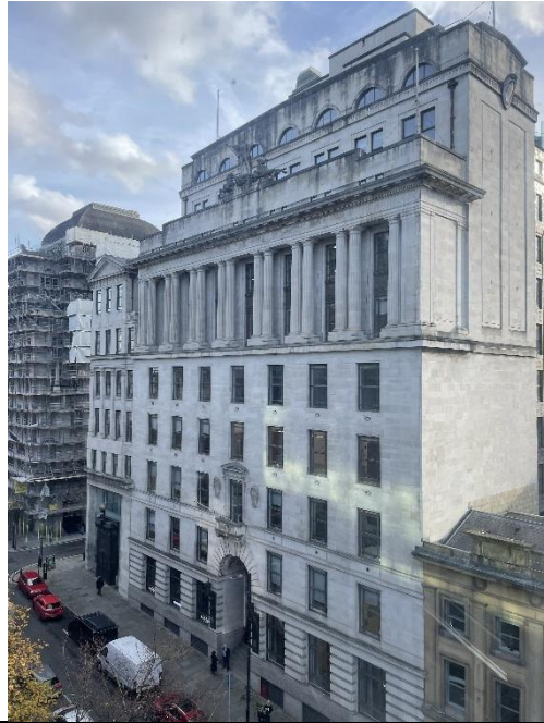
Figure 1 – Principal elevation of Ship Canal House (centre) and Atlas Chambers (left) fronting King Street. Source: Site Visit, October 2025.
