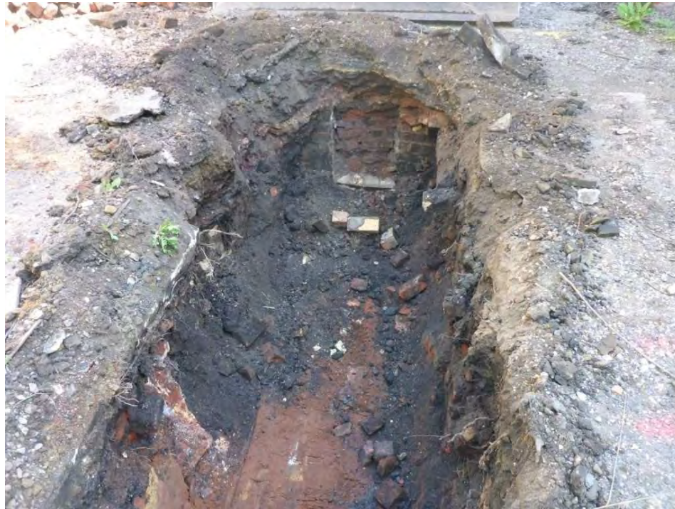
Trial Pit JTP30 - Photo 1
