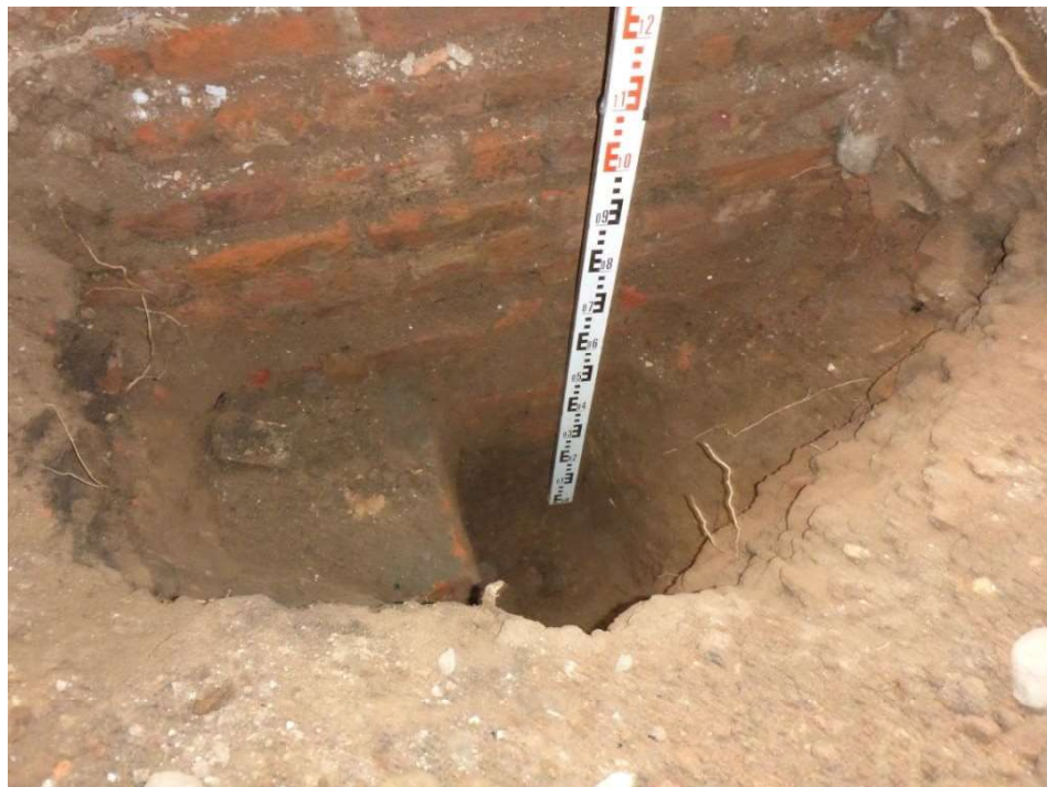
Trial Pit JTP12 - Photo 2
