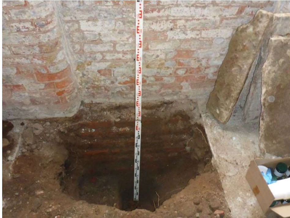
Trial Pit JTP12 - Photo 1
