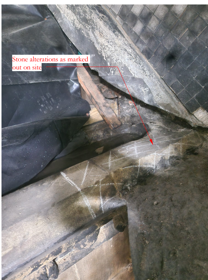
GHR04 - West Gutter South End
