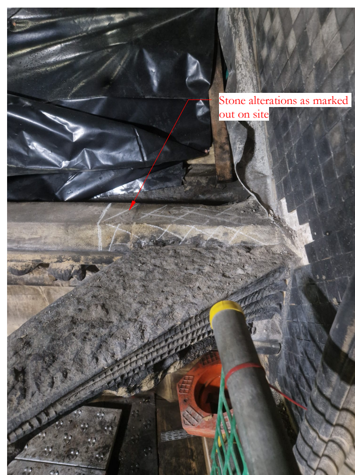
GHR04 - West Gutter South End
