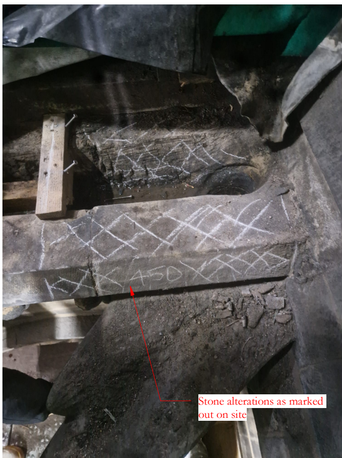
GHR03 - East Gutter North End
