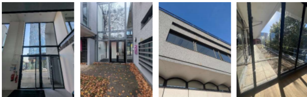
Existing Curtain Wall and Windows
