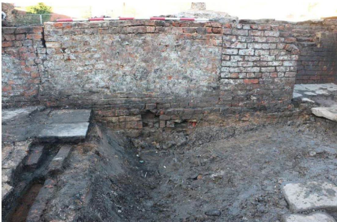
Plate 35: Original elements of the rear, north-western wall [166] left of shot, [166], looking north-west. Note the vertical phase break with remodelled wall [196] beyond. (scale: 2m)
