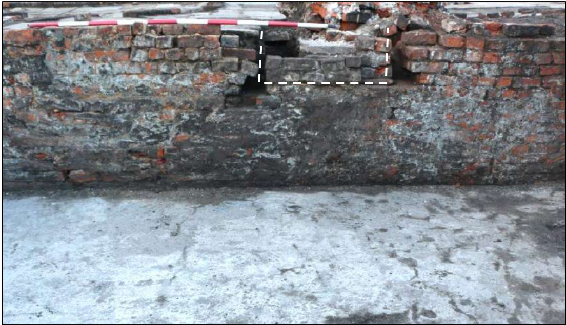
Plate 36: Rear wall [166] of cellar S2a with blocked cellar light [201]; looking north-west. (scale: 2m)
