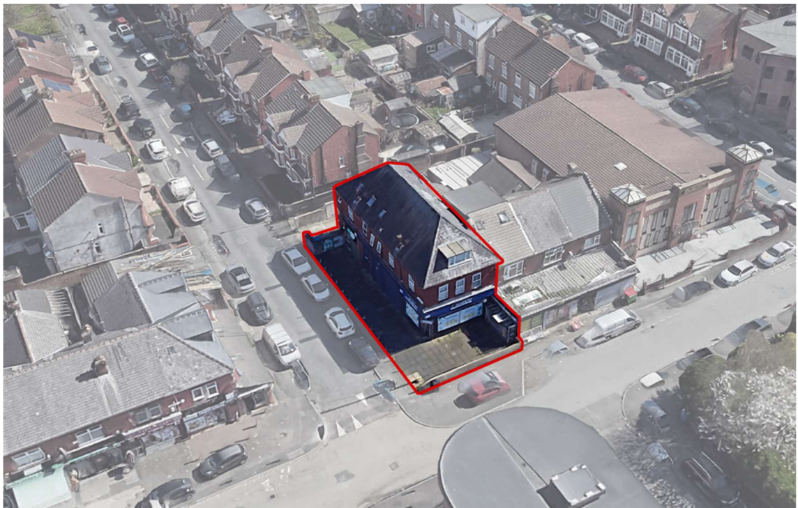
Aerial view to corner of site – the land ownership is edged in red.
