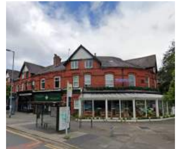
Corner building - 500 Wilbraham Rd
