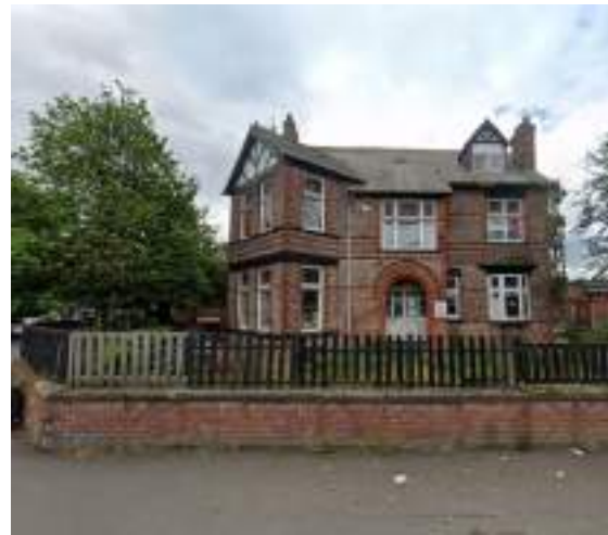
Existing building to be demolished
