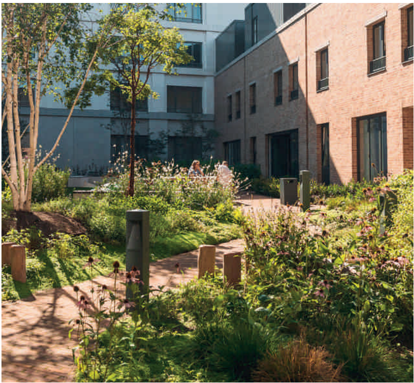
An attractive, south-facing landscaped area
