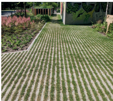
Reinforced grass paving
