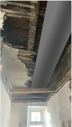
PHOTO SHOWING THE LOCATION OF VENT DUCT ABOVE WC WINDOW
