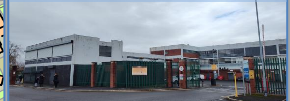
The western edge of the site and gated access to the rear, service yard
