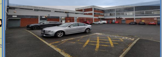
The service yard at the rear of the application site
