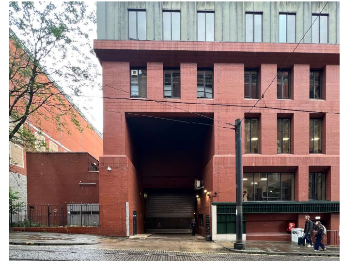
Existing compound and 1 Balloon Street loading bay adjacent (location of temporary chillers)
