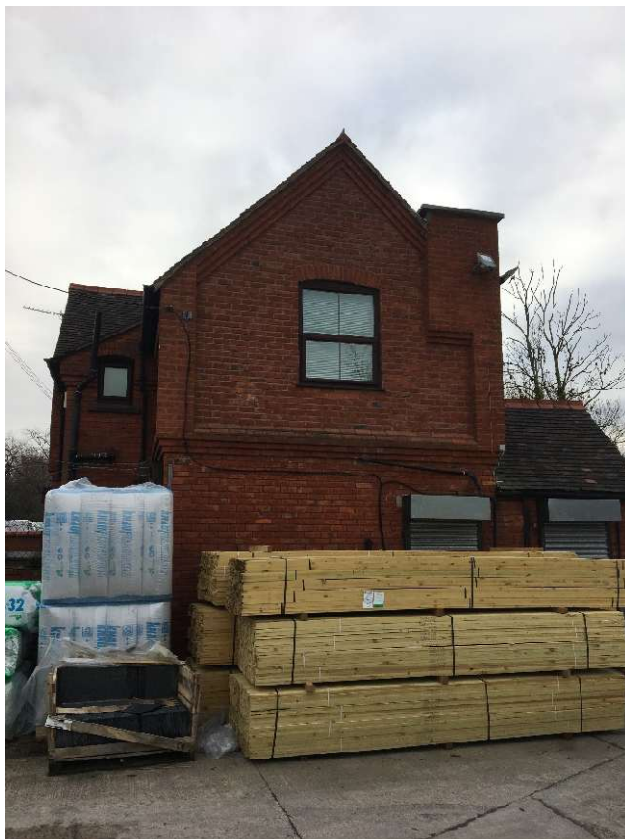
Side elevation to service yard
