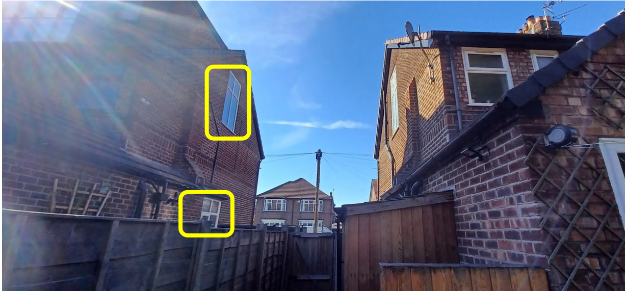
Figure 32. Side facing windows of No.41 Westholme Road
