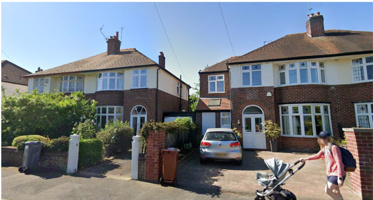
Figure 27. View of No.20 and No.22 Ferndene Road
