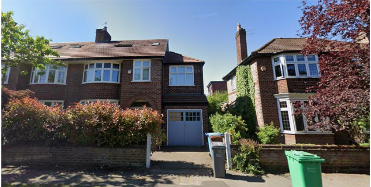
Figure 12. Existing side extension present at No.18 Westholme Road
