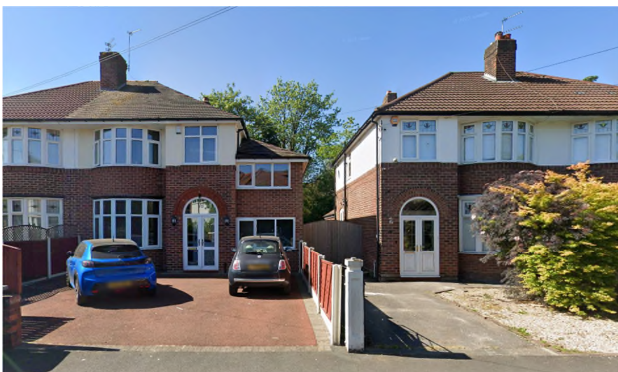
Figure 25. View of No.8 and No.10 Ferndene Road
