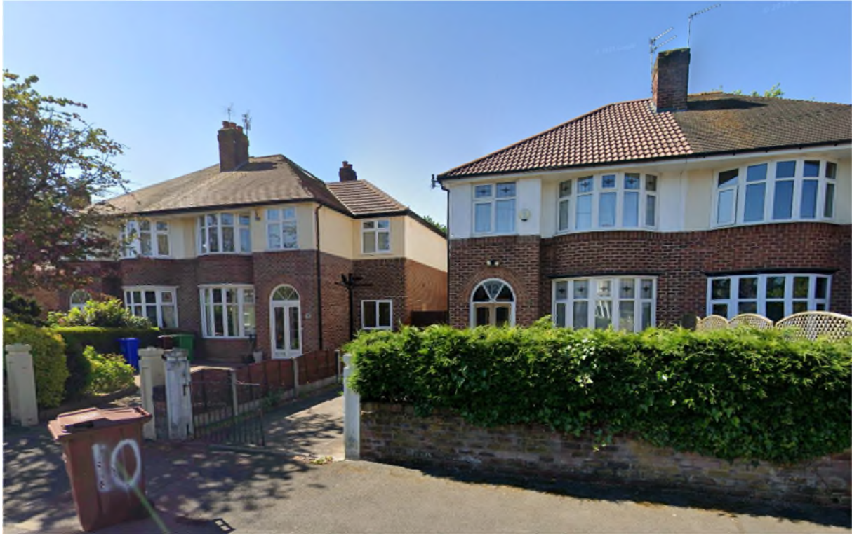
Figure 26. View of No.12 and No.14 Ferndene Road
