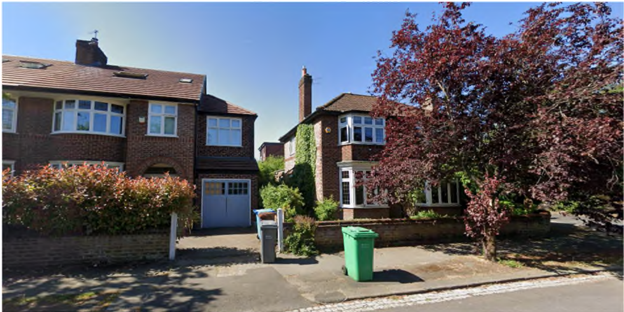
Figure 17. View of relationship between No.18 Westholme Road and No.1 Roseland Avenue
