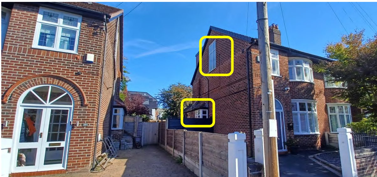
Figure 31. Side facing windows of No.41 Westholme Road
