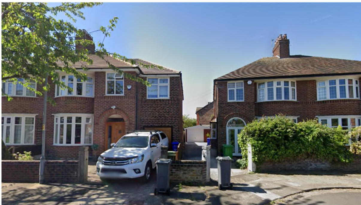
Figure 24. View of No.26 and No.28 Brooklawn Drive
