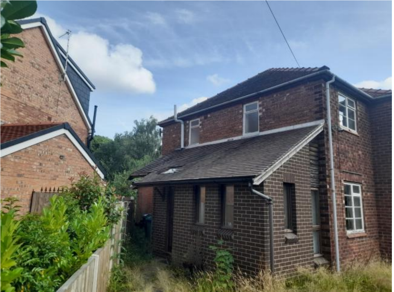
Application site – July 2022
