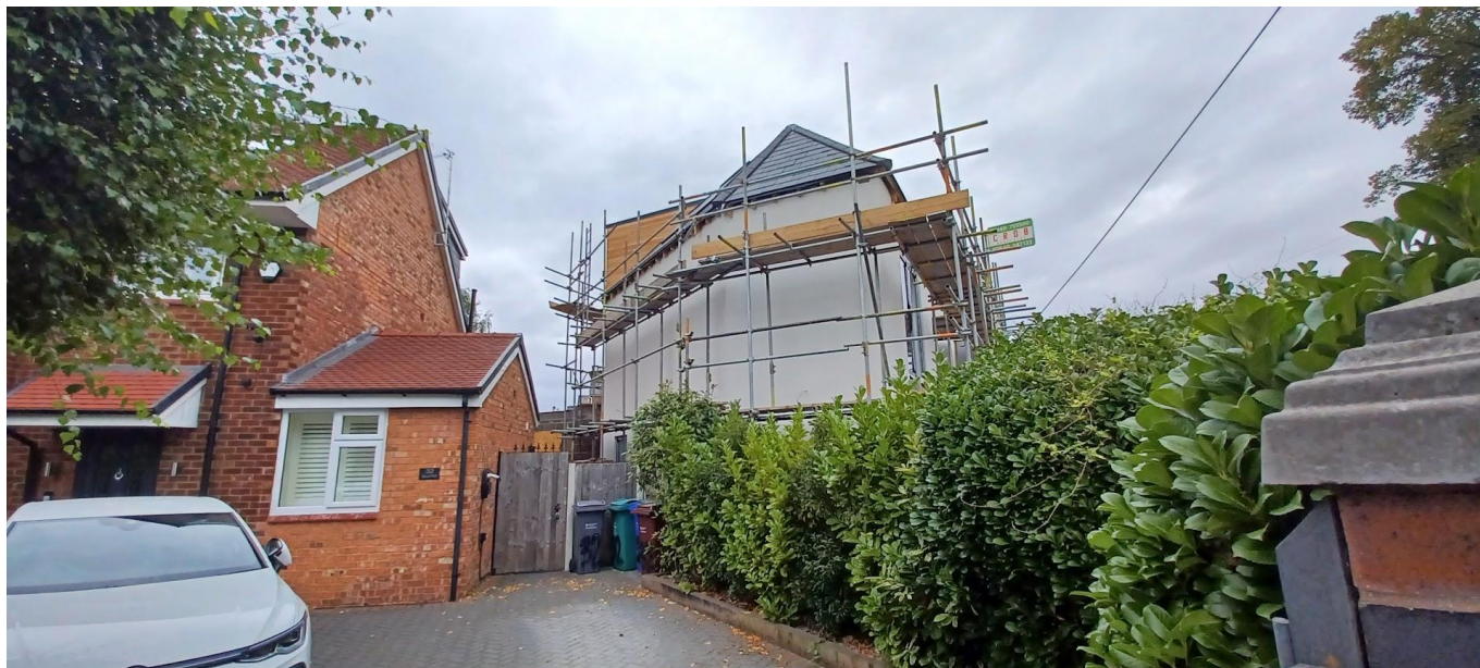
Side elevation of application property - August 2025
