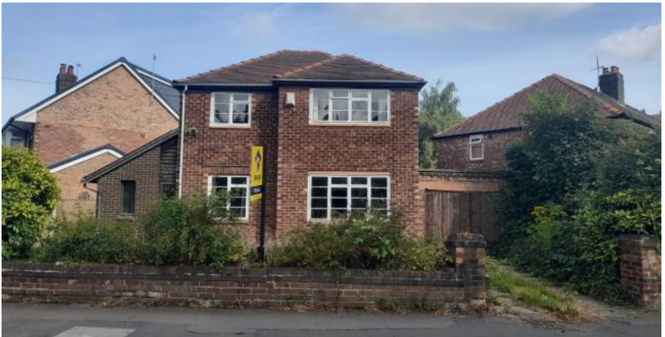
Application site – July 2022
