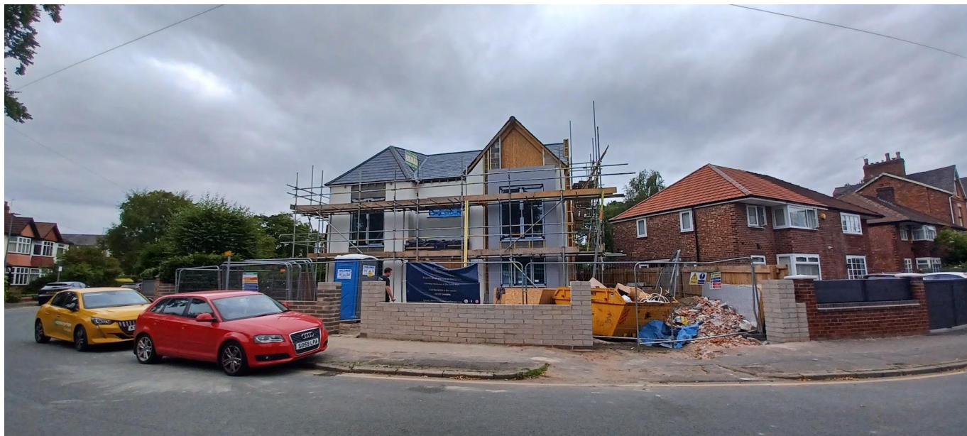
Street view of application property – August 2025
