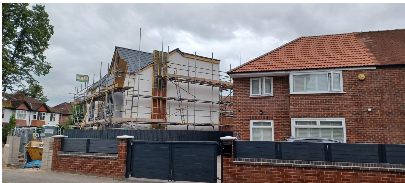
Side elevation of application property - August 2025
