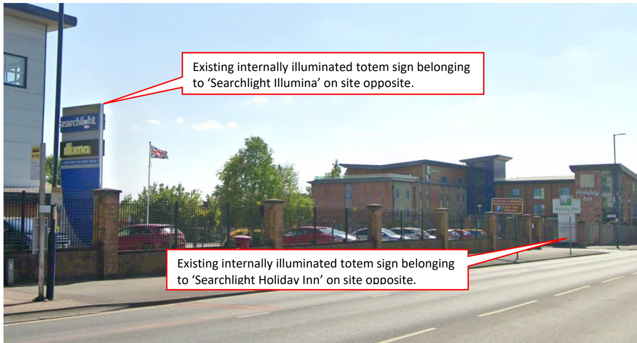
Image 5: Google Maps street view dated May 2025 indicating existing internally illuminated totem signage at Searchlight and Holiday Inn on Oldham Road opposite to the application site.
