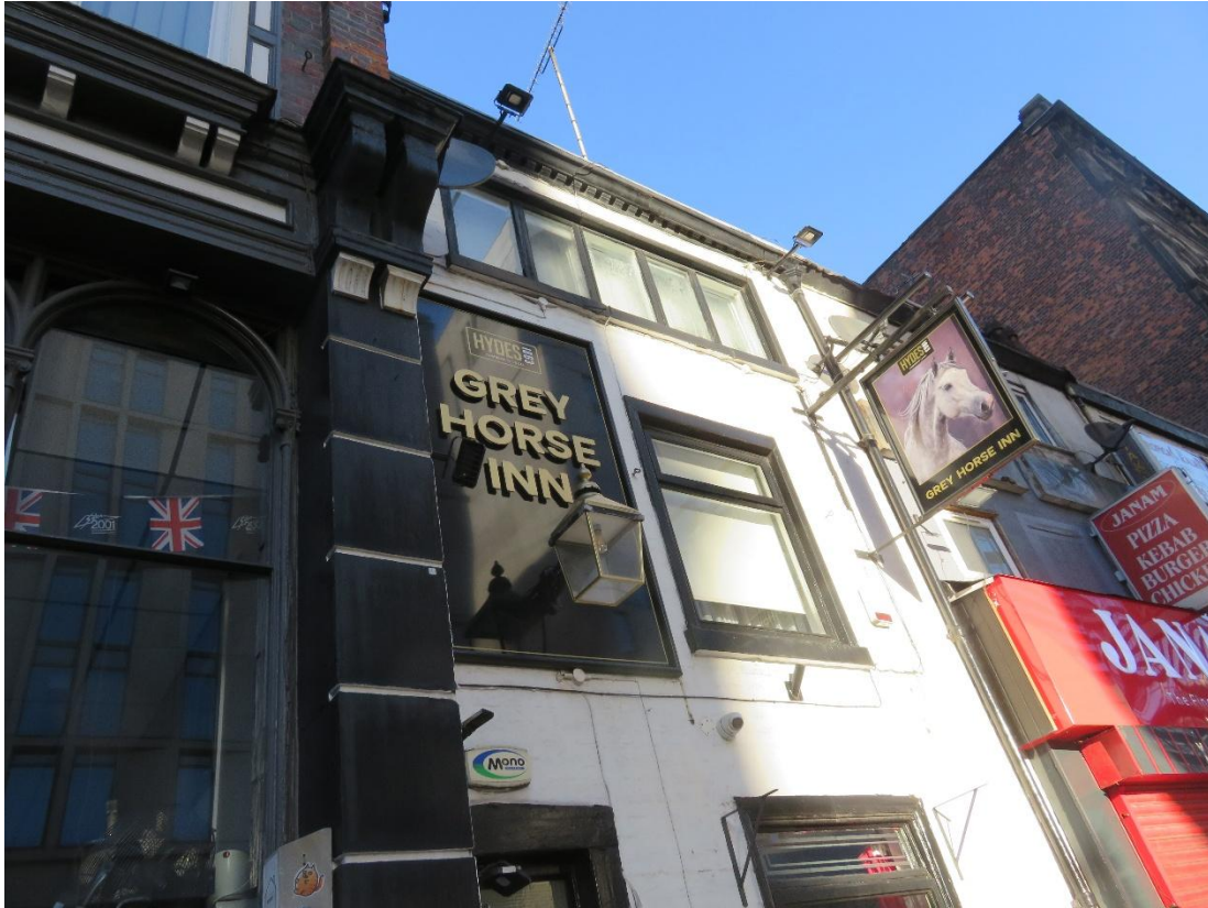
Second floor window possible use for weaving purposes.
