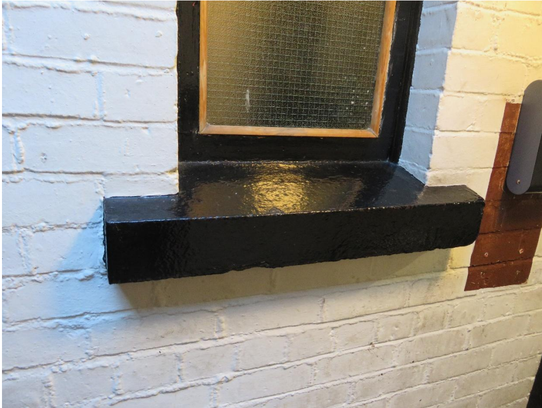
Chamfered 1900's window section with 225mm English garden bond brickwork.
