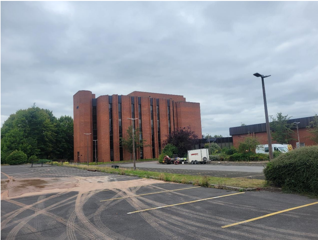
Plate B.5 Building 5 and car park which comprises of hardstanding and linear strips of grass and shrubs
