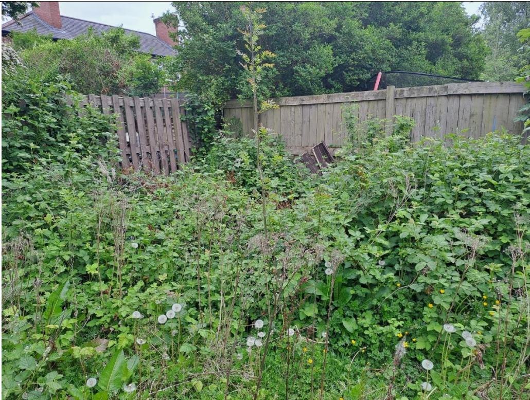
Figure 10: View of the southeastern corner of the site.
