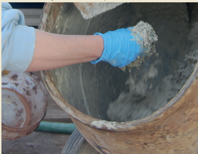
Assessing the workability of the lime hemp plaster and deciding whether or not to add water
