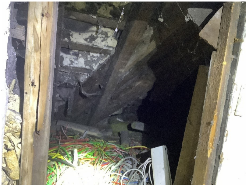
Figure 17 Visible loft interior
