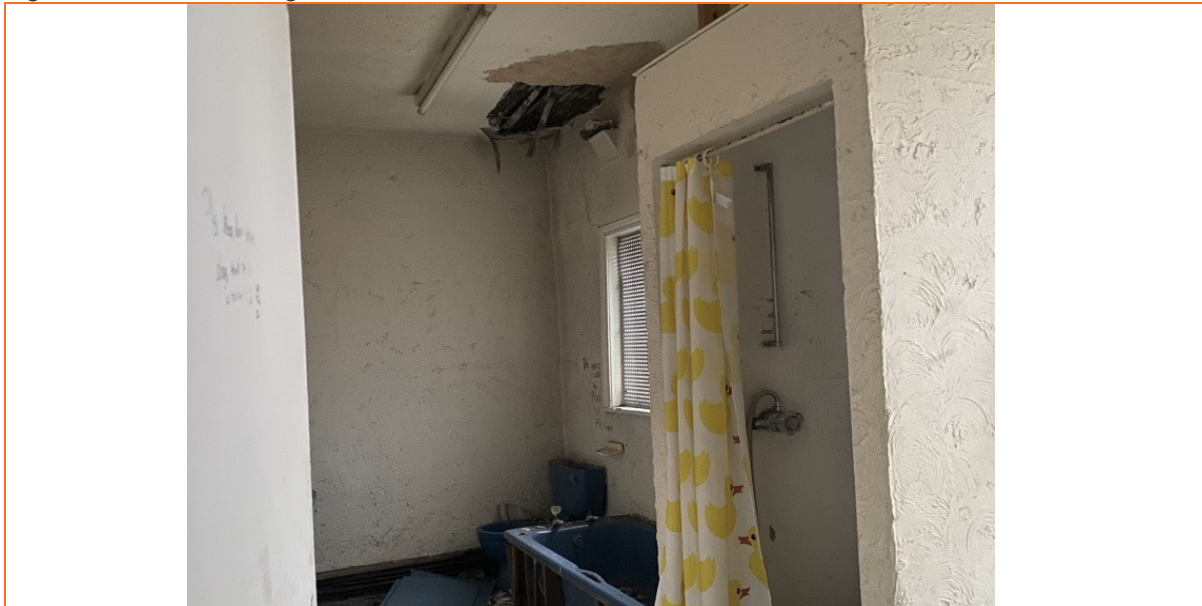
Figure 11 Showing Ground Floor
