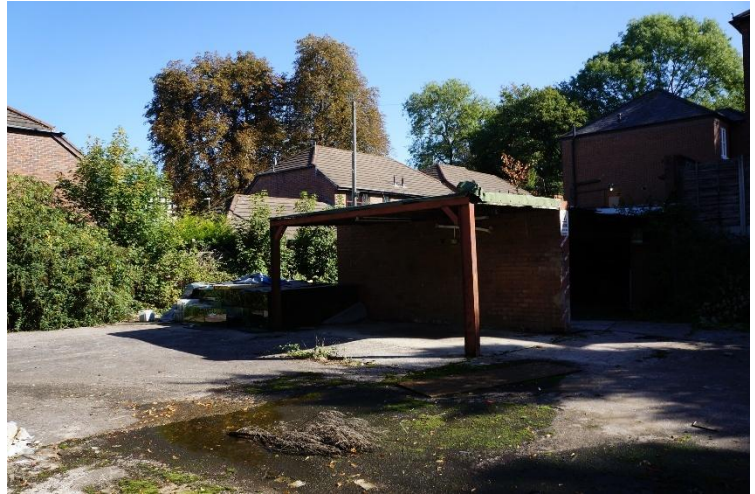
Figure 4: B1 Building and concrete hard standing.
