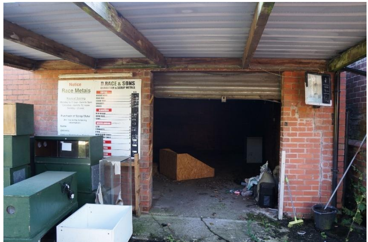
Figure 12: Entrance to the garage section of the building.
