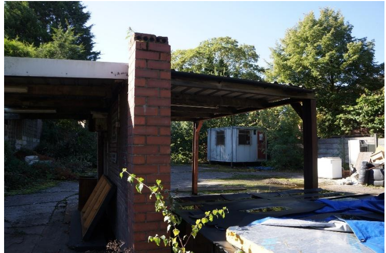
Figure 10: Open carport style extension to the building.
