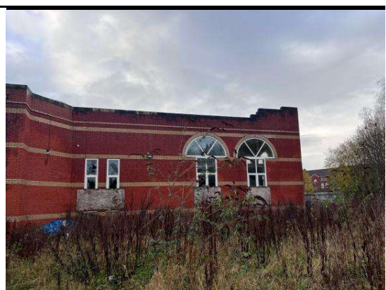
Photo 4: View looking west towards the disused mosque building with overgrown vegetation in the foreground
