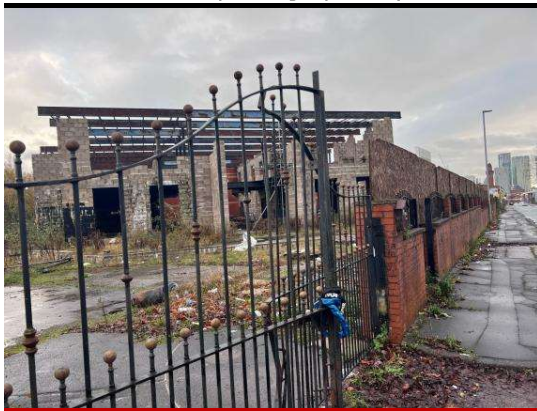
Photo 1: View of the gated site entrance from Sherborne Street, showing the brick boundary wall and existing abandoned building within the site
