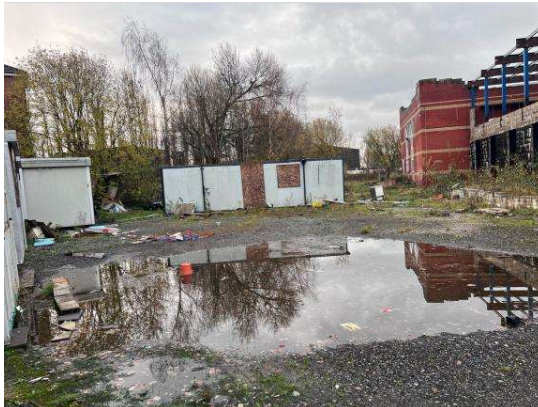
Photo 5: View of surface water ponding in the northern part of the site, indicating poor infiltration and limited existing positive drainage
