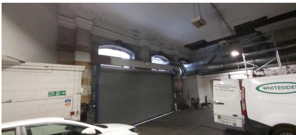
Photo 3. Former Clerks Room, now a service area/car park, showing roller shutter door to Milk Street, plaster boarded ceiling and plant extracts. Original Internal decorative marble piers are visible on rear wall. Remnants of the glazed rooflight remain above the new ceiling.
