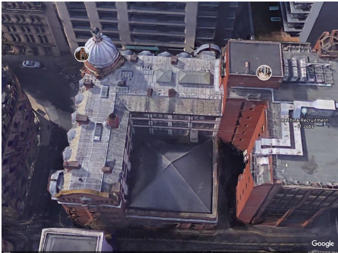
Figure 2: Google aerial photo showing the three storey L-shaped office chambers and the pyramid roof above the service yard on Milk Street. The York Street entrance to the offices (3 York Street) is bottom left near the junction with Milk Street and the entrance to the Brasserie is top left under the dome at the junction with Spring Gardens
