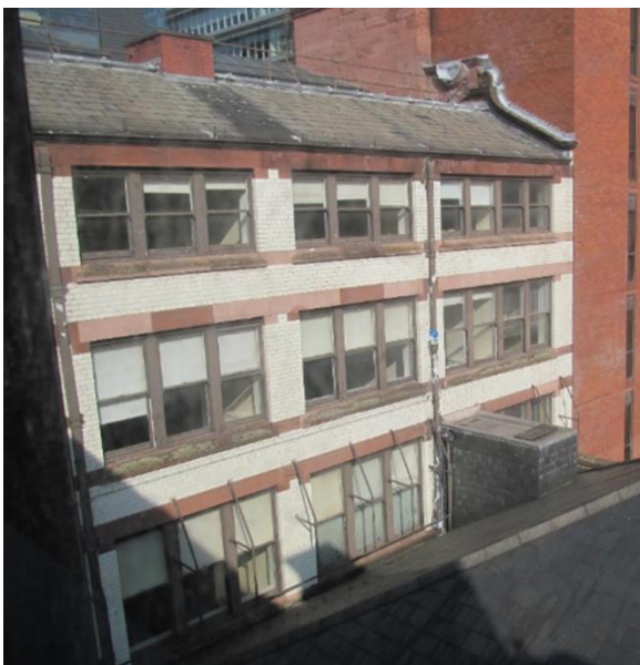
Photo 9. Upper floors of offices having a modest low-key design to the rear of service area. 30304 casements under a slate room and white reflective tiles.
