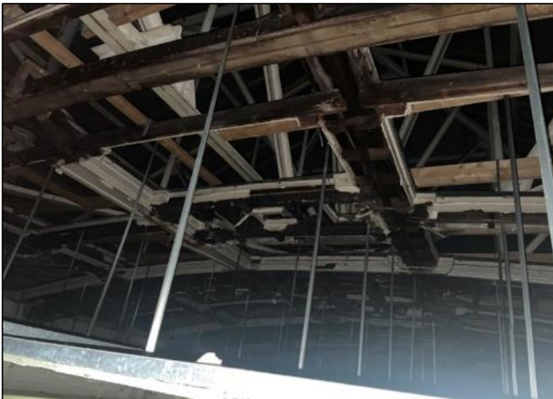
Photo 14. Support structure of domed ceiling over the Clerks' Room, with the new pyramid shaped slated roof above and hanger supports for the ceiling of the service yard
