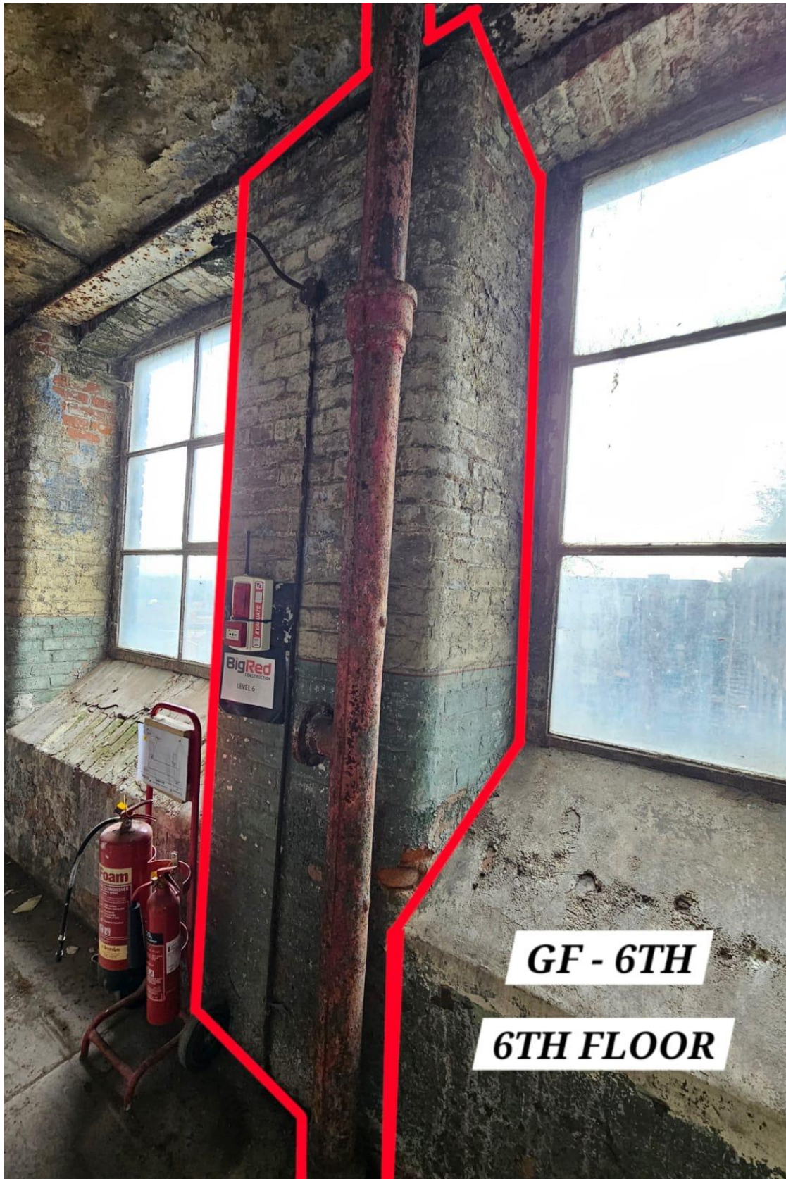
West staircase - 6th floor. Early 20th century painted floor level sign for “No 7 Spinning Dept”. The red outline denotes the extent of paint retention, which includes the pier from floor to ceiling, both returning reveals to either side, and the late-Victorian/Edwardian vertical red fire sprinkler pipe.
