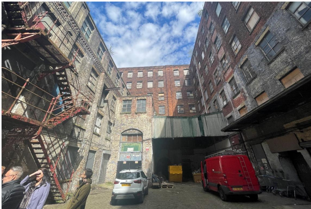
Looking north across the central courtyard, illustrating the lower levels of the exterior masonry that requires paint removal.
