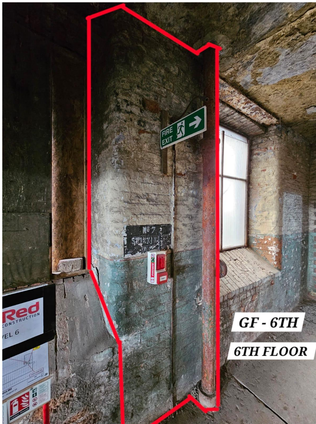
East staircase - 6th floor. Early 20th century painted floor level sign for "No 7 Spinning Dept". The red outline denotes the extent of paint retention, which includes the pier from floor to ceiling, both returning reveals to either side, and the late-Victorian/Edwardian vertical red fire sprinkler pipe.
