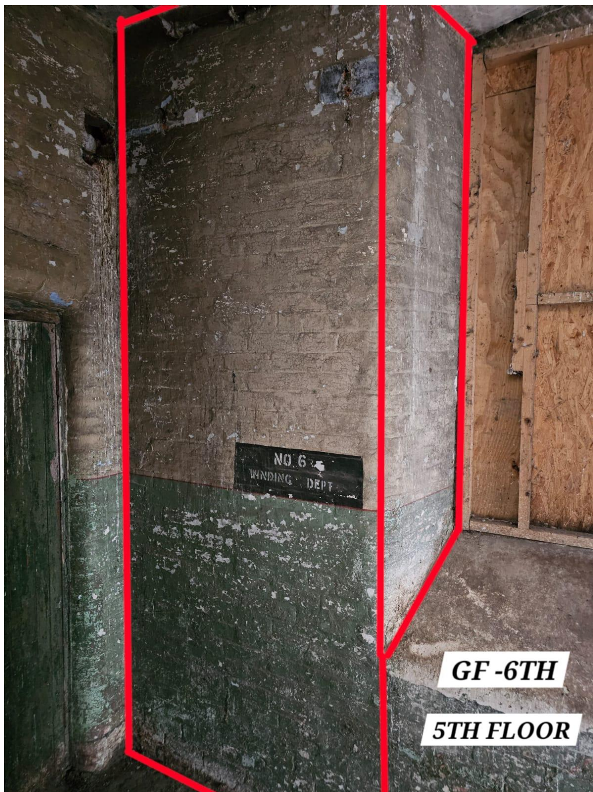
West staircase - 5th floor. Early 20th century painted floor level sign for “No 6 Winding Dept”. The red outline denotes the extent of paint retention, which includes the pier from floor to ceiling and returning reveal to the window side.
