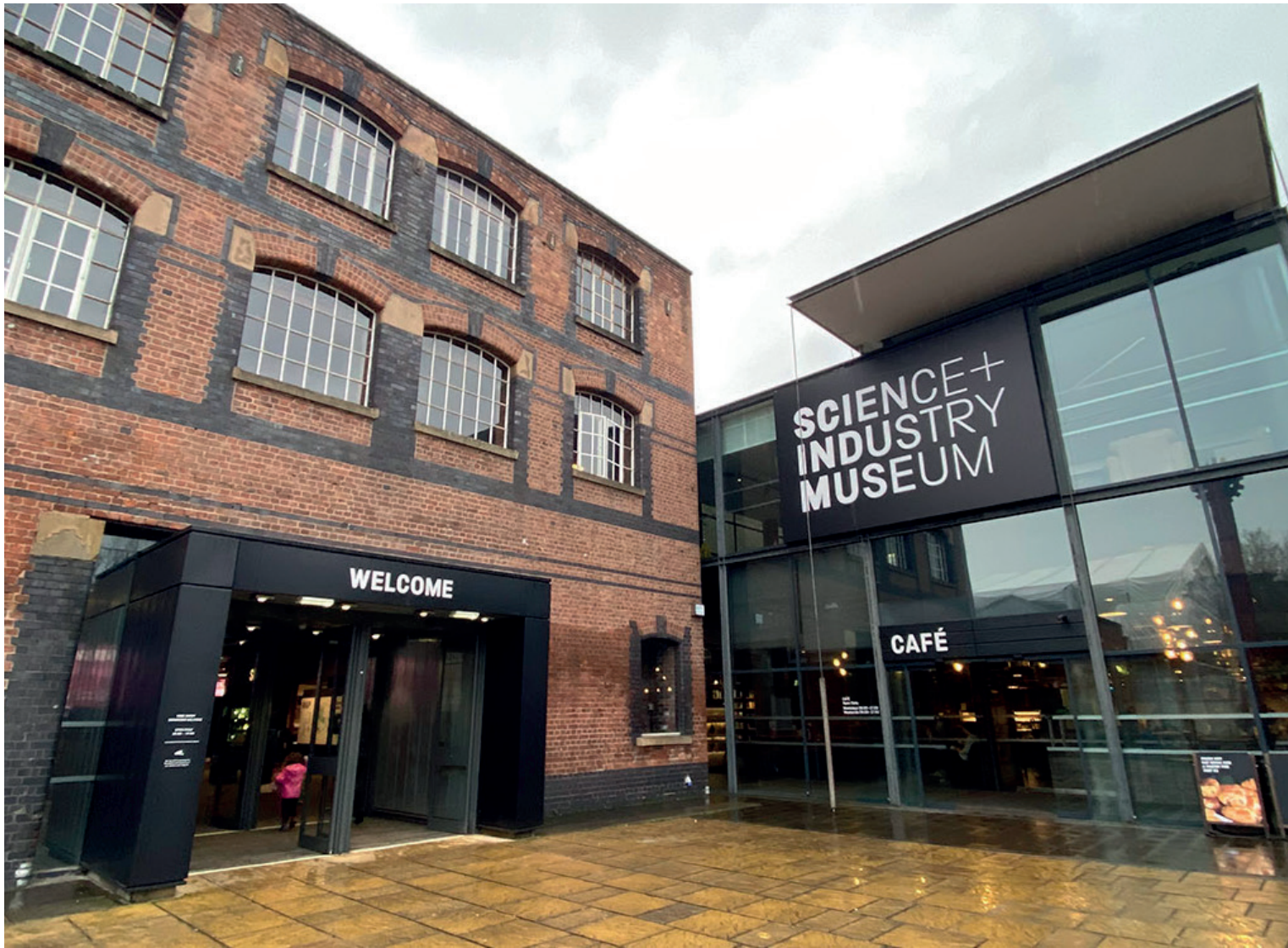
Image: External view of New Warehouse.
