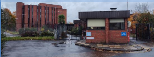
The gatehouse and Brotherton House seen from the entrance to the site on Cornfield Drive
