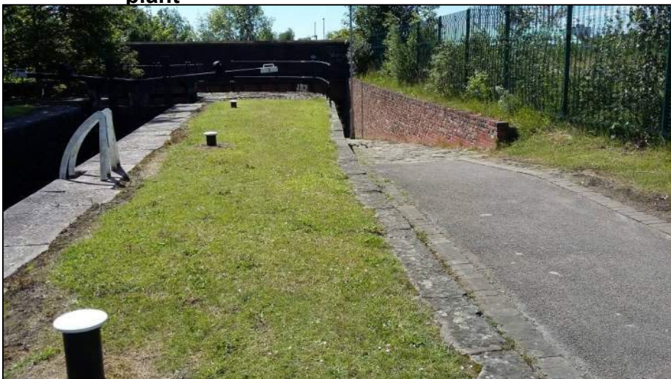
Photo 12 Bridge across the canal, looking west and unimproved neutral grassland verges
