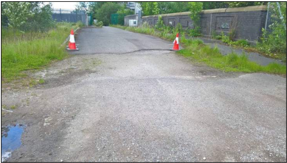
Photo 1 Tarmac road over canal bridge, accessing the site from the south
