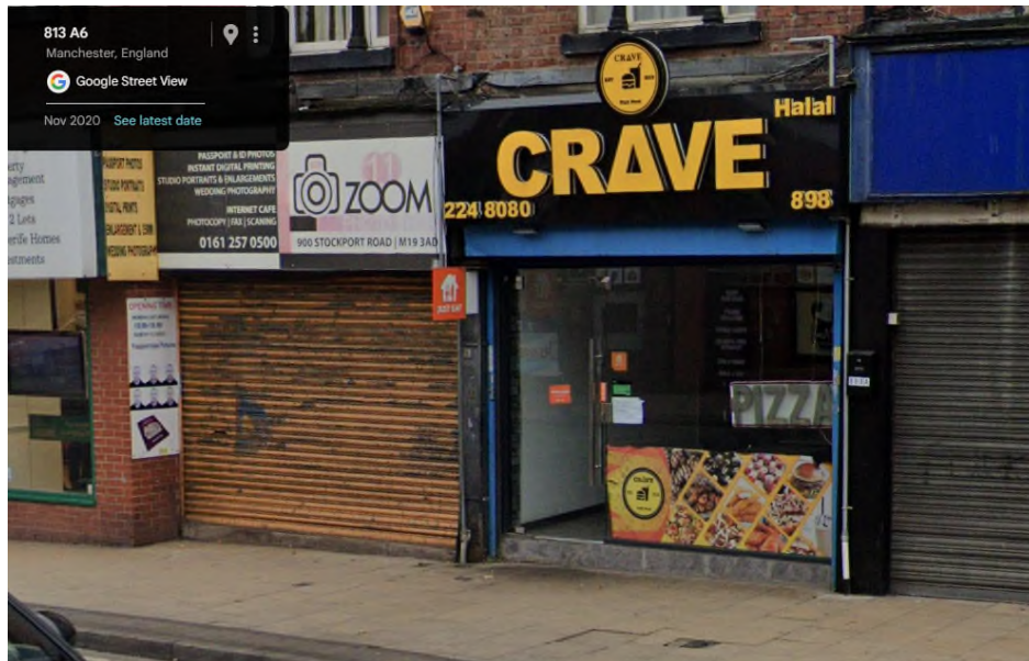
Fig.3 – Application site in November 2020
