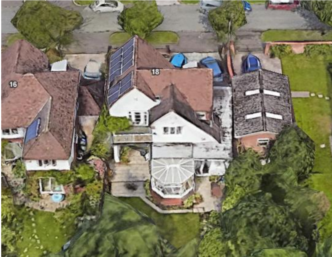
Rear view of No.18 Sussex Avenue
