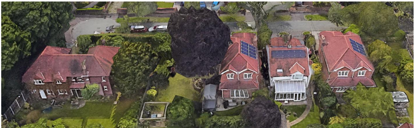
Rear view of No.5b-d and No.7 Sussex Avenue
