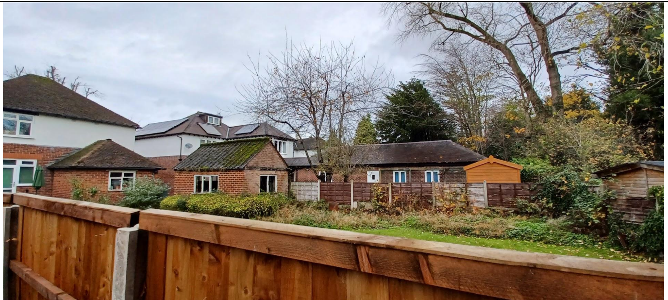
View of large outbuildings in neighbouring gardens
