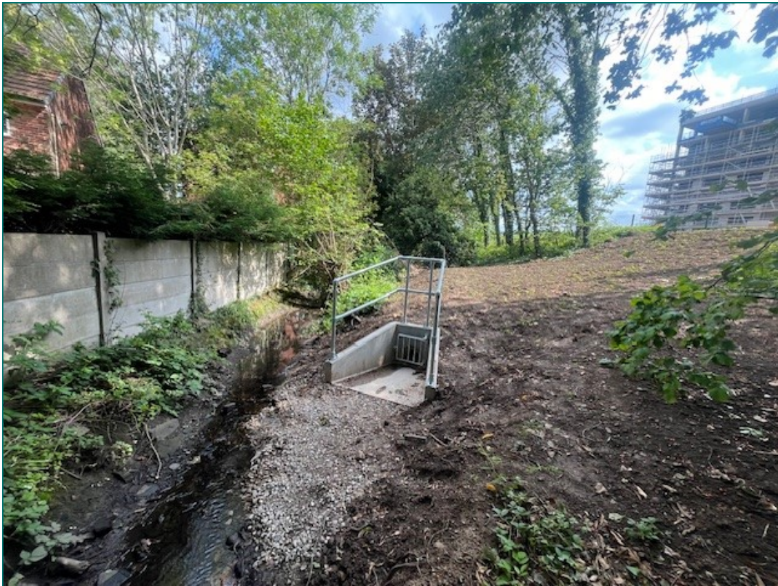
Photograph 4 Headwall Installation.
