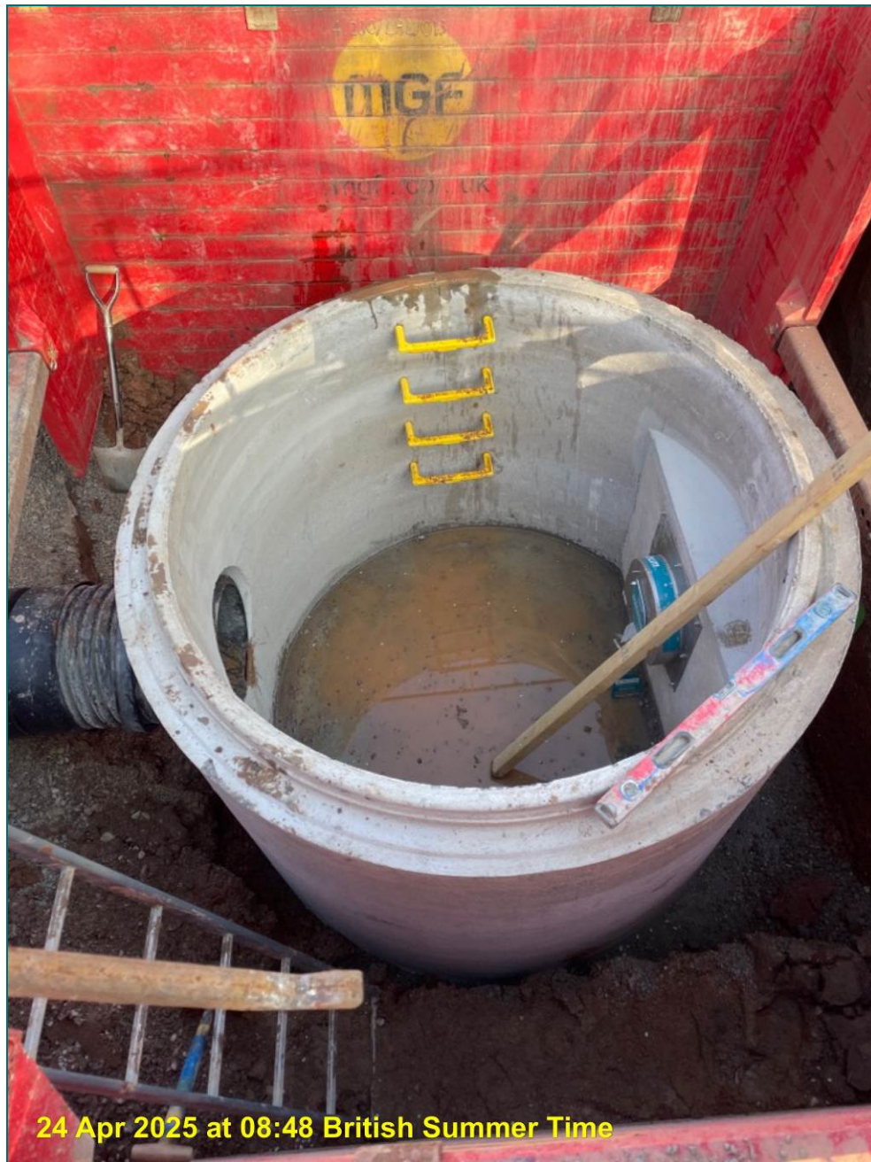
Photograph 3 Flow Control Installation
