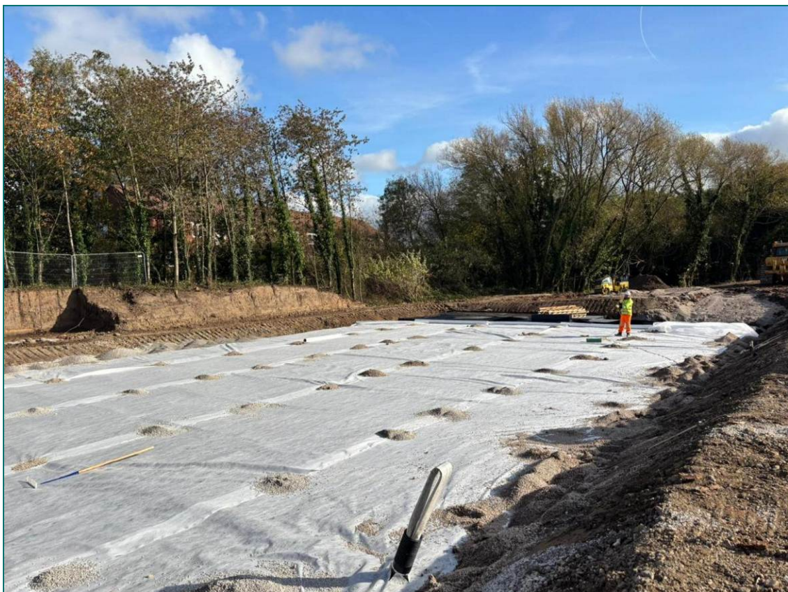
Photograph 2 Attenuation Installation
