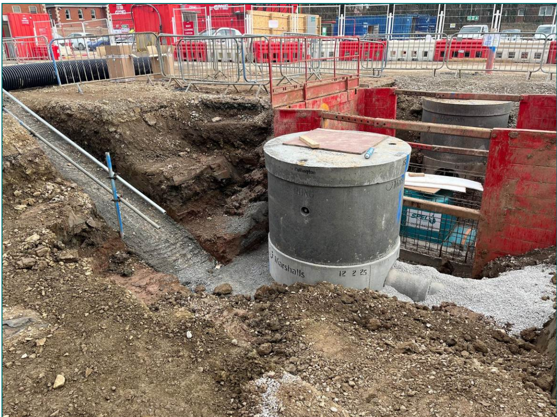
Photograph 5 Interceptor Installation.
