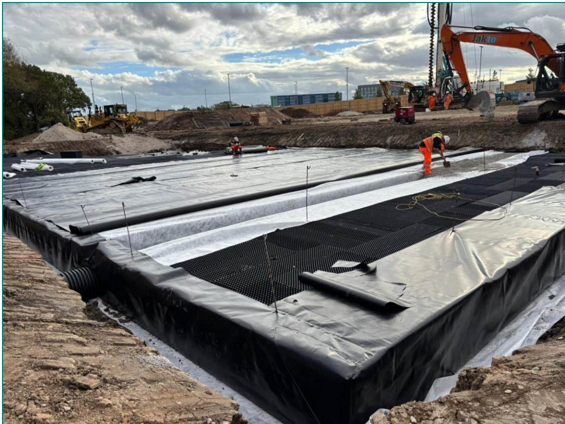
Photograph 1 Attenuation Installation
