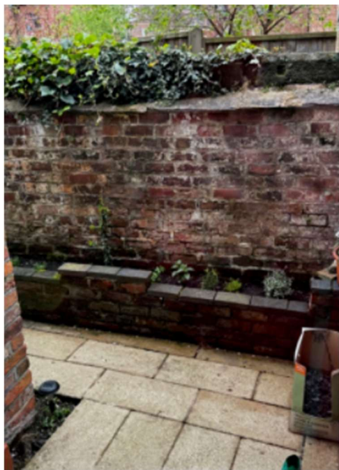
View of a section of existing wall
