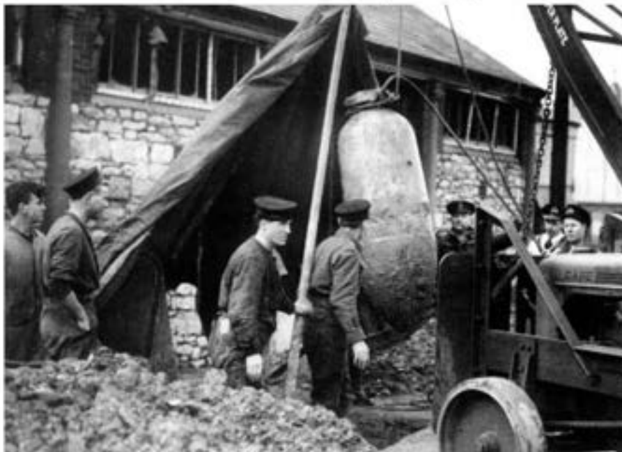
Removal of an UXB
