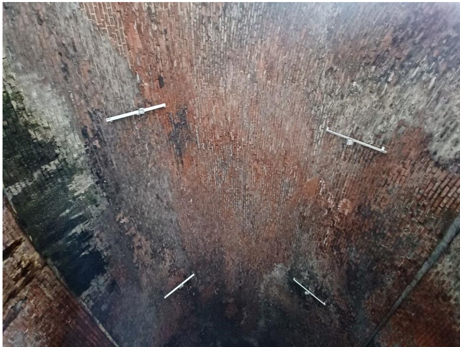
Photo 6: General view of span 1 soffit looking north to south.
