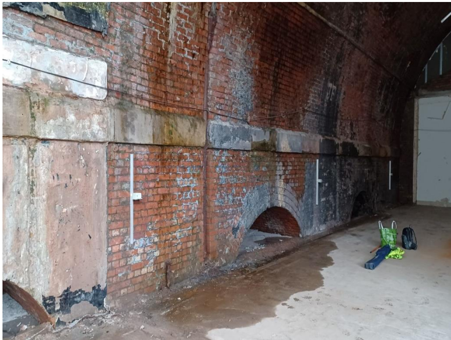
Photo 8: General view of west face of central pier showing relieving arch.
