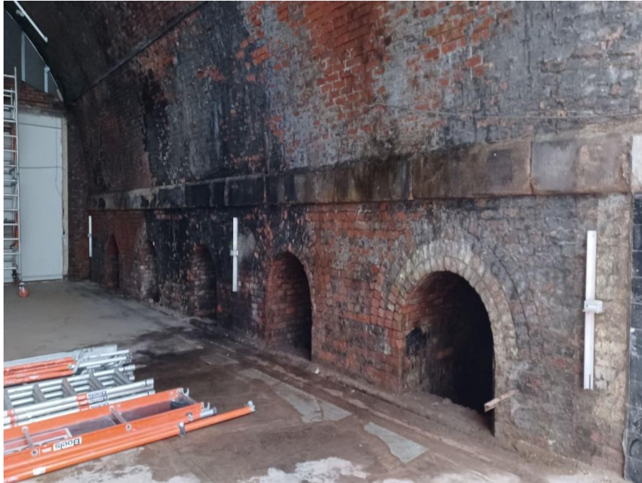
Photo 7: General view of west abutment showing relieving arches.
