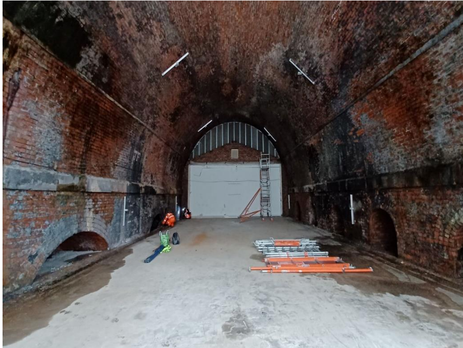
Photo 5: General view through span 1 looking north to south.
