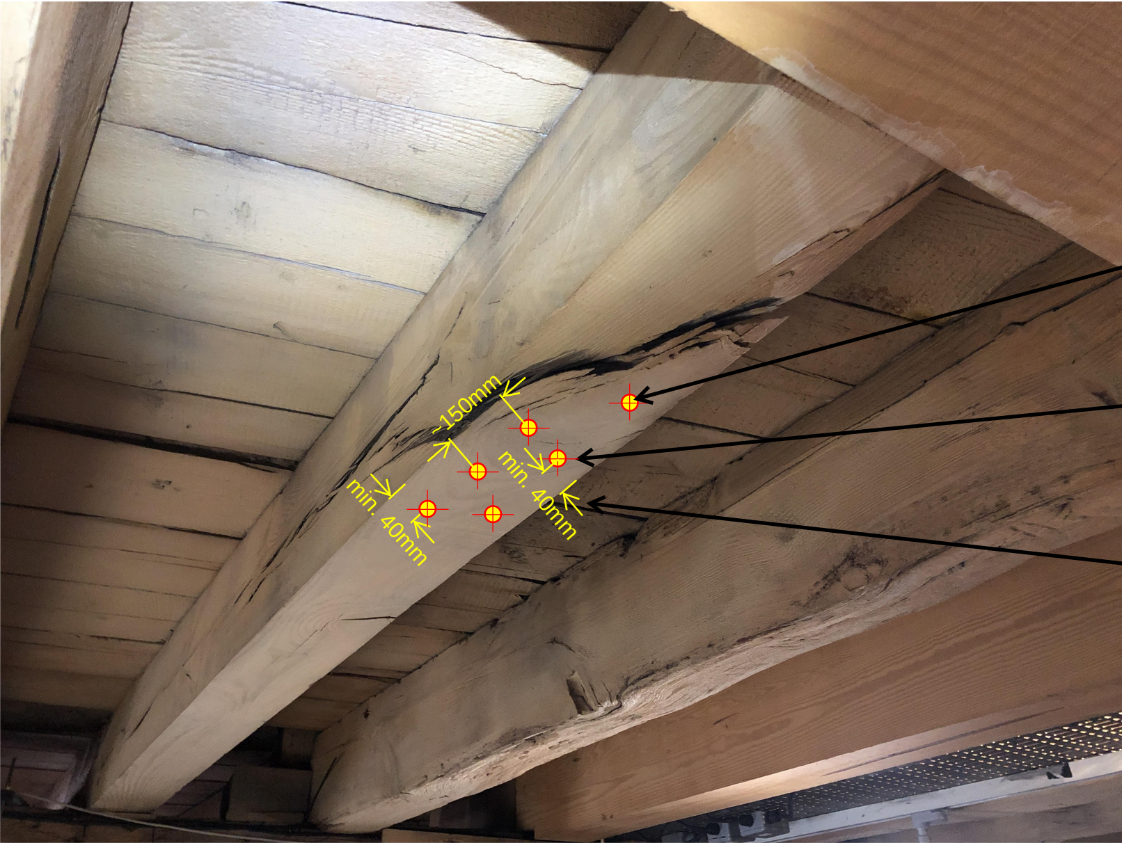
FIGURE 1: FIXINGS - TYPICAL SETTING OUT & SPACING AT UNDERSIDE
