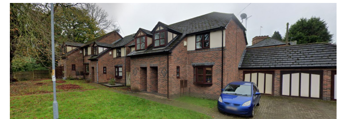
Above: Modern housing located on Ollerton Close which is located off Boat Lane.
