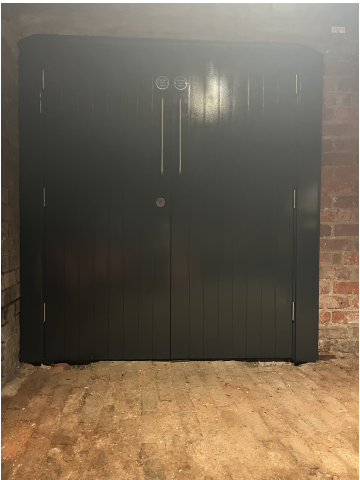
Locally slightly raised cobble finish
