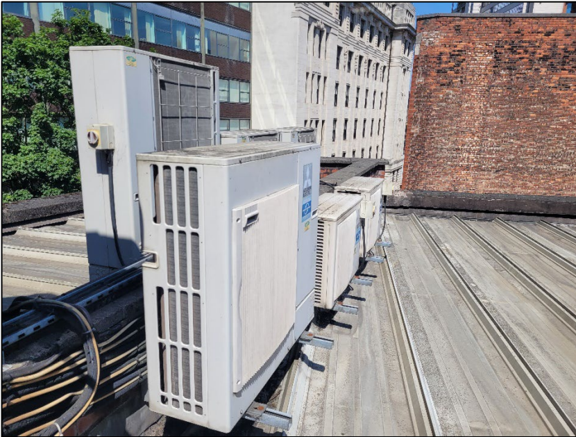
Photograph 4 Southern structure at roof level
