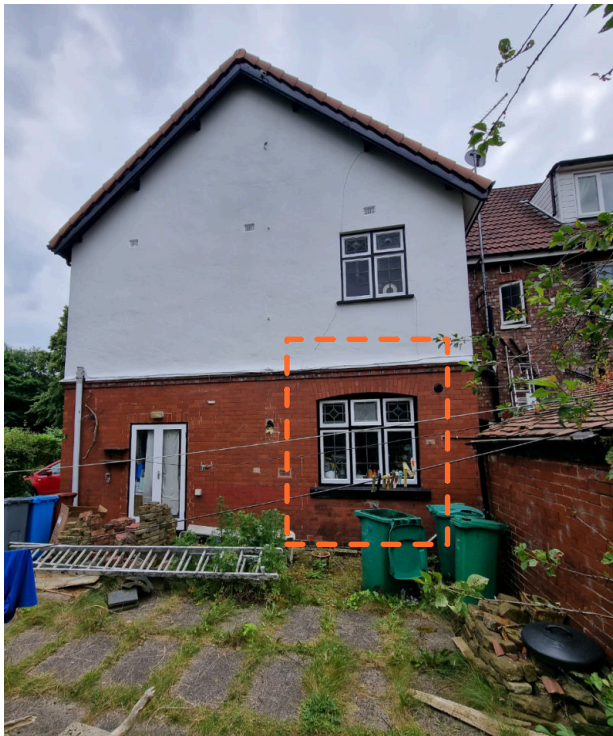
Existing kitchen window to be re-used in east porch
