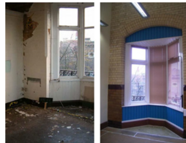
2.3.42 Transit Room before (c.2000) and after (c.2008) refurbishment(Todd)
