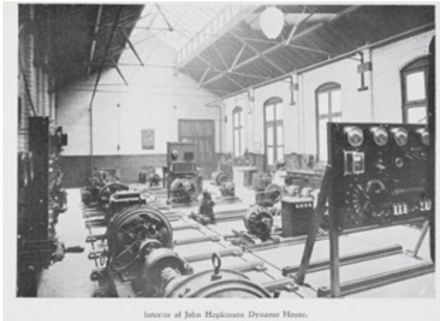
2.3.6 Dynamo House (ground floor), 1906
