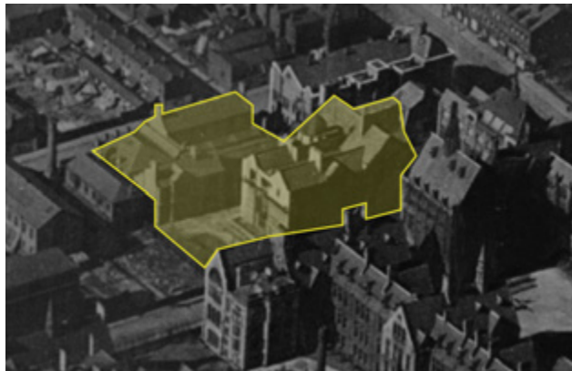
2.3.34 Main building and John Hopkinson annexe, c.1925 (University of Manchester)
