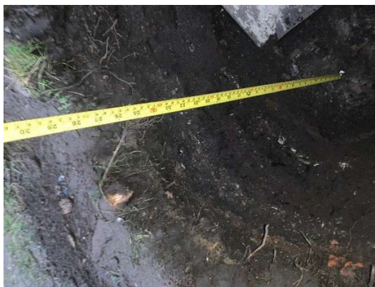
Photographs of Trial Pit indicating Stiff Clay at 0.65m Depth
