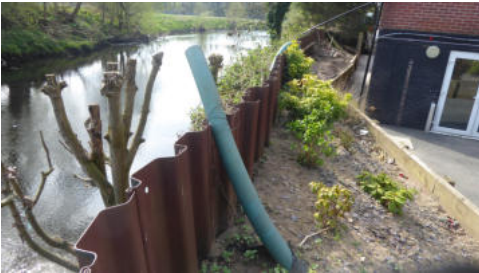
Figure 1.2: Sheet Piled Wall
