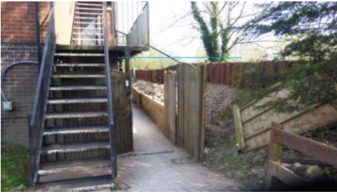
Figure 1.1: Sheet Piled Wall
