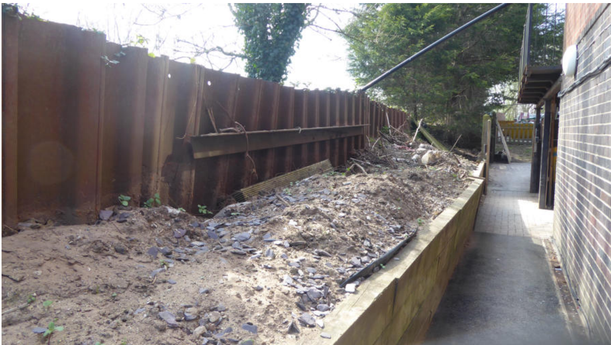
Figure 1.3: Sheet Piled Wall
