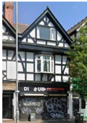
Figure 1 Street view of site
